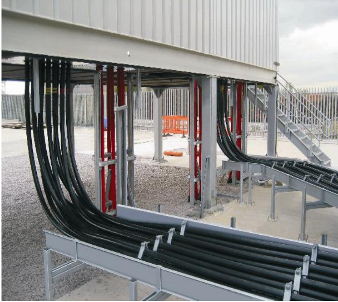
Fig. 5. Example of a power cable assembly in a conductive cable tray.
