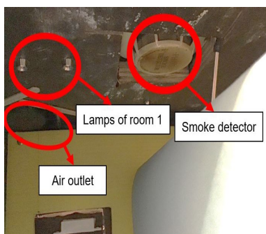
Fig. 14. Lamps in room 1, smoke detector, and air outlet of the simulated house.
