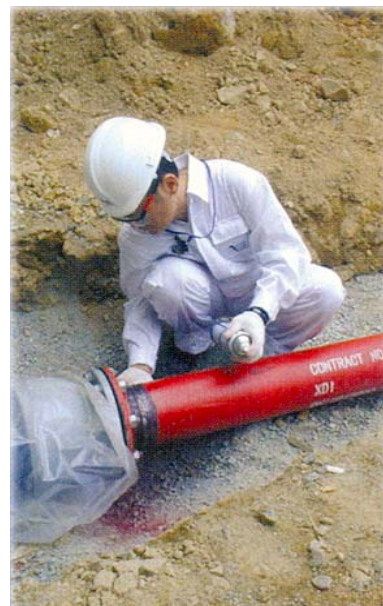
Figure 4: Working posture of an inspector during performing DPI (Source: ETS-Testconsult Ltd.)
