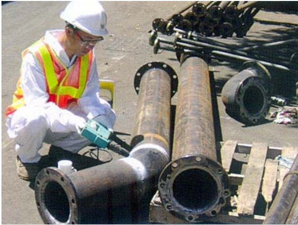
Figure 5: Working posture of an inspector during performing MPI (Source: ETS-Testconsult Ltd.)
