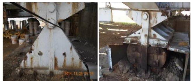
(a) fixed support (b) sliding support Fig 2. Photographs of trestle supports
