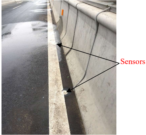
Fig. 4. Data sensor installation of the road
